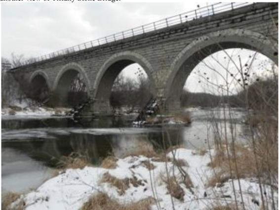
The safety chain guard railing was replaced in 1935 with a pipe railing. During the 1930's a steel mesh covered with concrete was cast inside the arches to improve load carrying ability. The typical road engine today weighs about five times that when the bridge was built. The bridge is 387 feet long by 16 feet wide and supports a single track.
